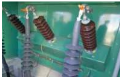
The 3M™ Cold Shrink Termination QT-III for 69kV is designed for indoor and outdoor installations.
